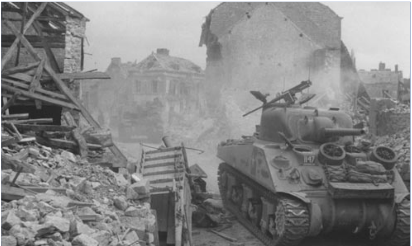
XXX Corps advancing through a badly-damaged French village in August 1944
